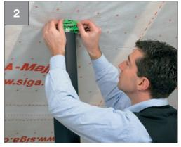
Apply Rissan half to the pipe and half to the vapour control layer without tension
