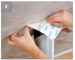
Remove the slitted backing strip from the centre out
