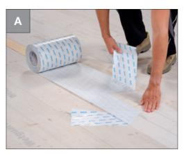
Bond element connecting joints e.g. butt boards etc. with Wetguard 390 mm
