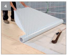
Remove the backing strips, unroll Wetguard and press firmly onto the substrate with a brush or surface wiper
