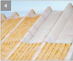
Fill insulation material in compartments in a tight fit
