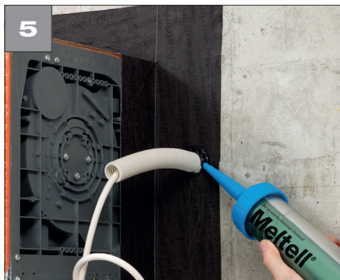
Penetrations • e.g. cable penetrations
