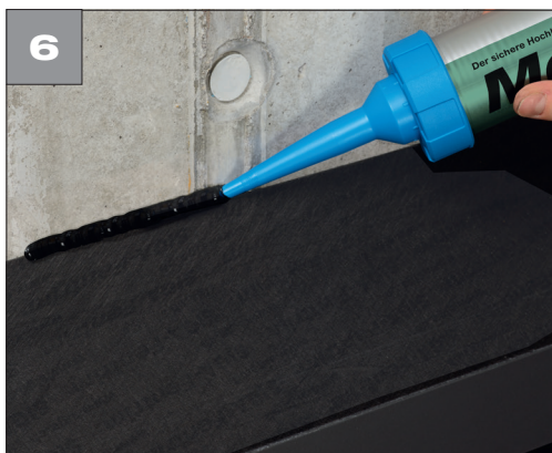
• Cracks, joints, imperfections
