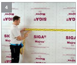
Seal overlap with Sicrall avoiding tension and wrinkles
